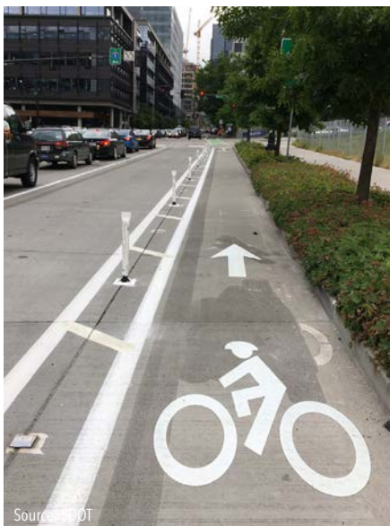
Use of paint and simple vertical features can provide safety benefits at a lower cost and with faster implementation.
