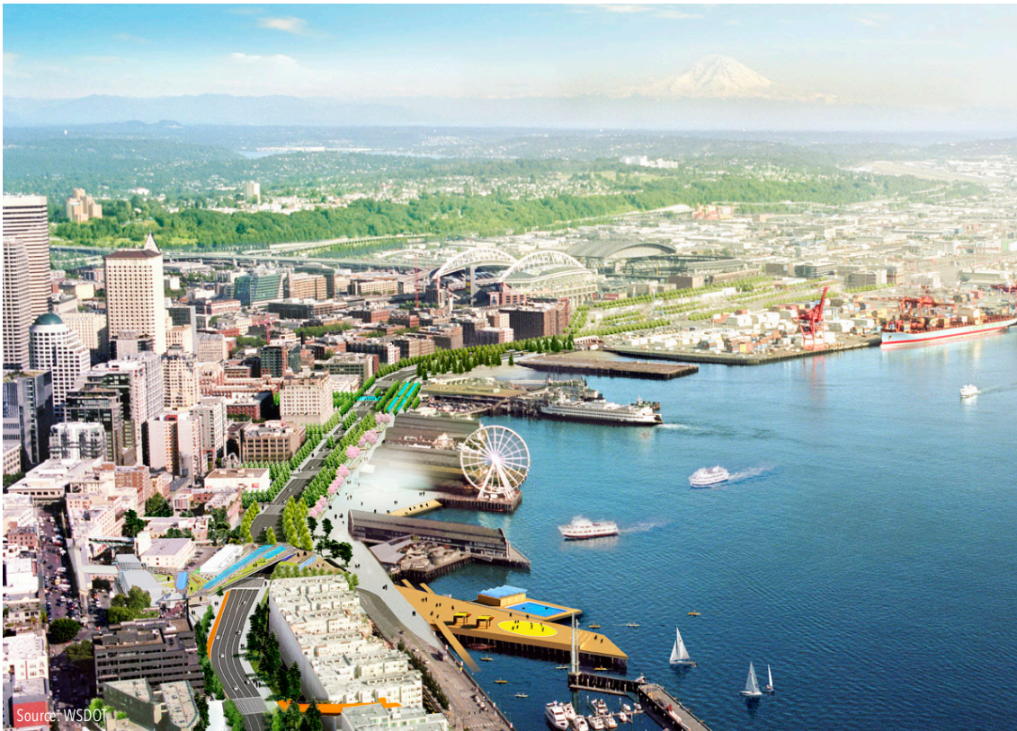
A rebuilt Alaskan Way will reconnect downtown Seattle to the waterfront.
